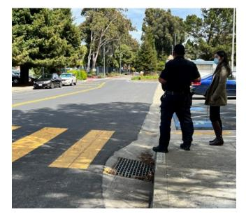
**Figure 17.** A view of the storm drain that prevents construction of a curb ramp on the south end of the crosswalk.
